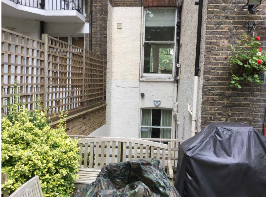
View of Infill Extension Location
