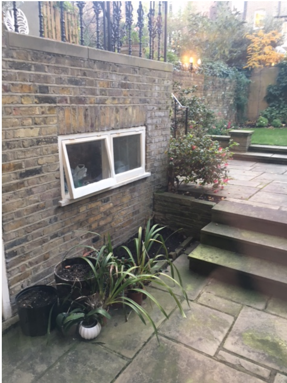
Affected basement level window at 46 South Eaton Place, with a reduction in VSC of 28%.
