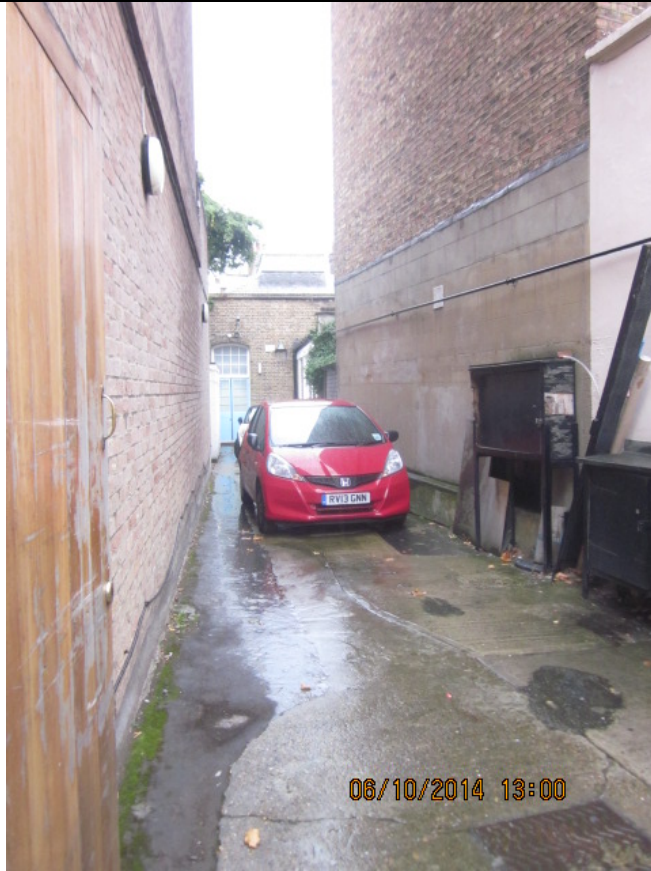
View of rear of Morison Building from passageway on Ebury Street
