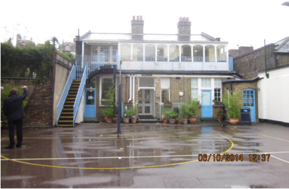
View of Northern elevation of Morison Building
