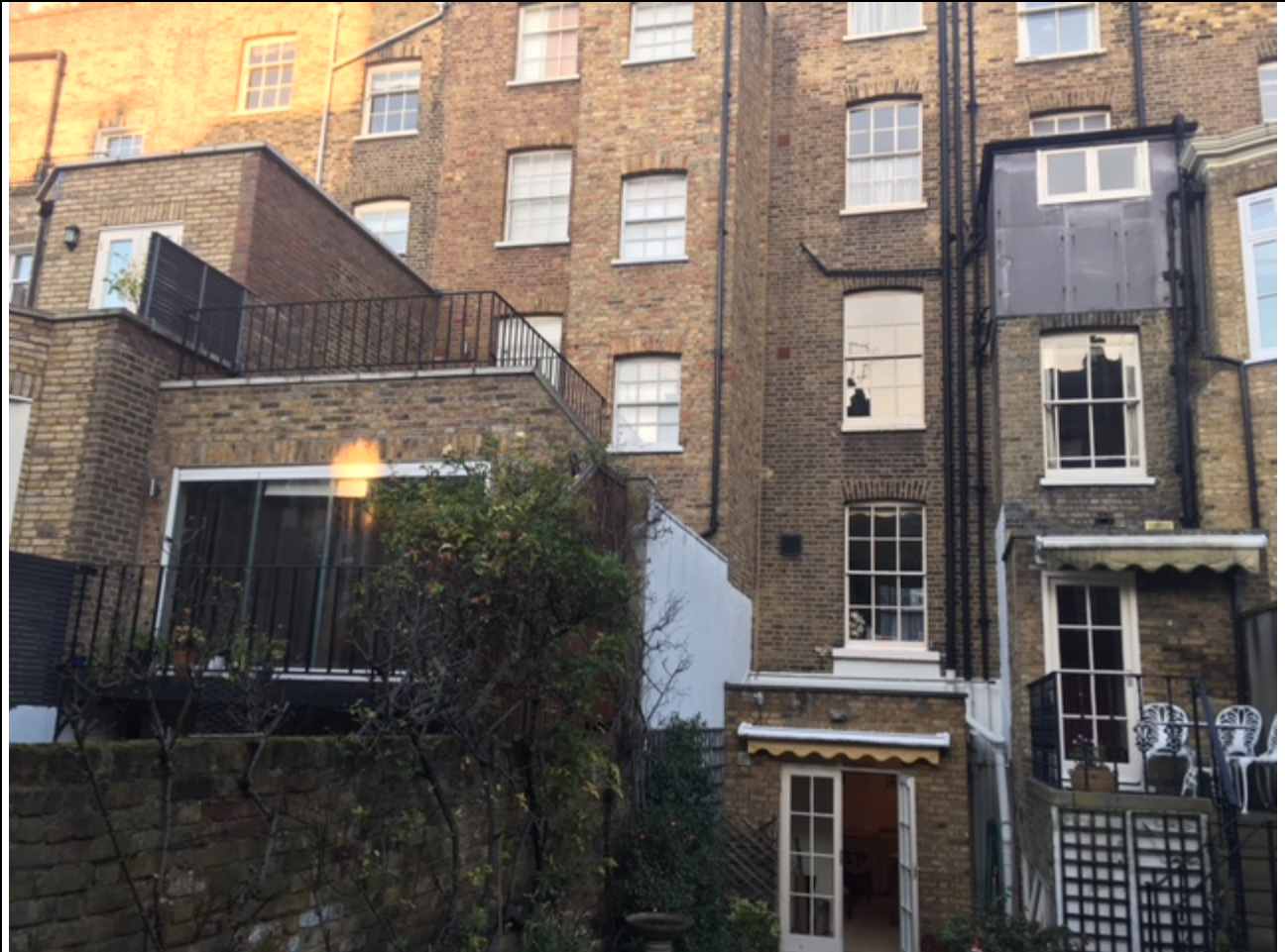
Rear elevation of 44 South Eaton Place (taken from neighbouring rear garden at 46)
