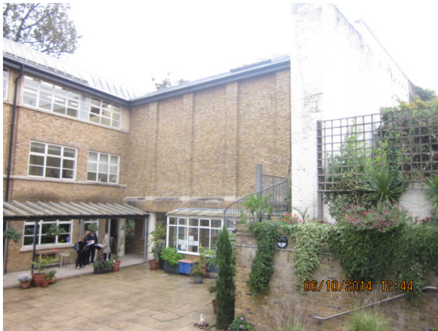
View of Grosvenor building
