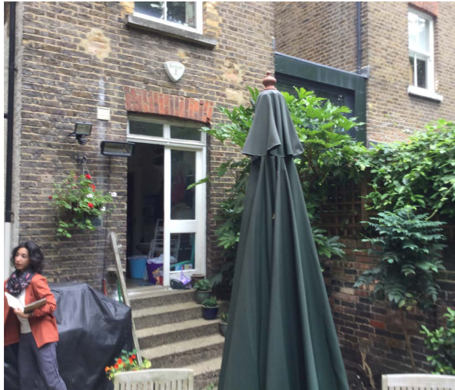
Rear of Existing Closet Wing
