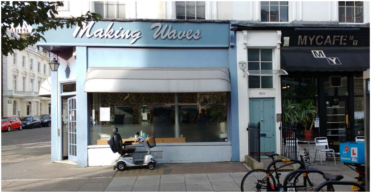
Nos. 95 and 93 Charlwood Street
